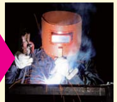
Resume welding works.
